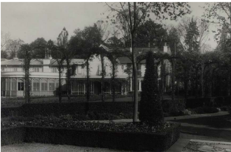
Figure 8: The Gardens at James Hazen Hyde’s Estate at Versailles. Source: ‘France, ca. 1932. James Hazen Hyde gardens, designed by Hazen Hyde to surround his 19th-century estate, near Versailles. View of house and garden.’ Bonney, Therese. 1925. Therese Bonney photographs, 1925-1937., Smithsonian Libraries, https://library.si.edu/image-gallery/91019
